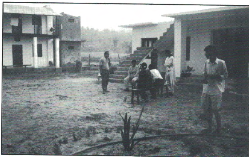
Complex of Women's training institute of WOREC at Rajabas, Udayapur. Parts of training building (right) and Dormitory (left)
